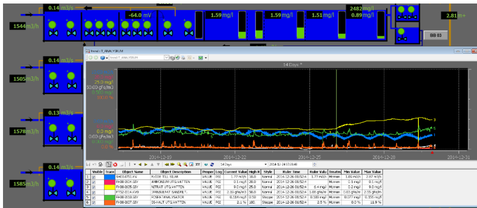
Figure 2. Example of the DCS 800xA 5.1 controlling all equipment at the Käppala WWTP and surrounding facilities.
